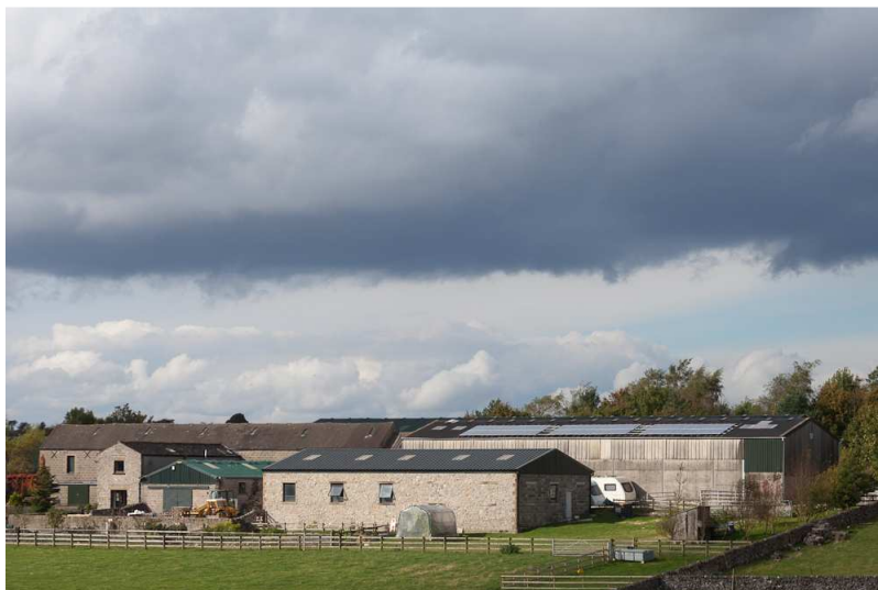
Photo 5. Solar Photovoltaics, Shallow Grange Farm
