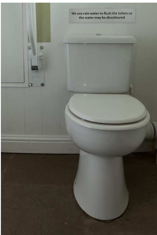
Figure 13 Rainwater harvesting for toilet flushing
