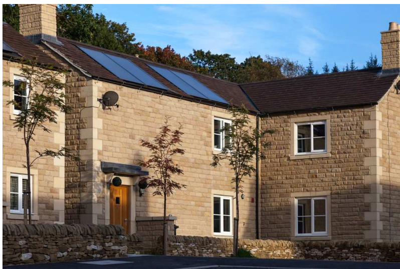
Photo 3. New build affordable housing, Bamford
