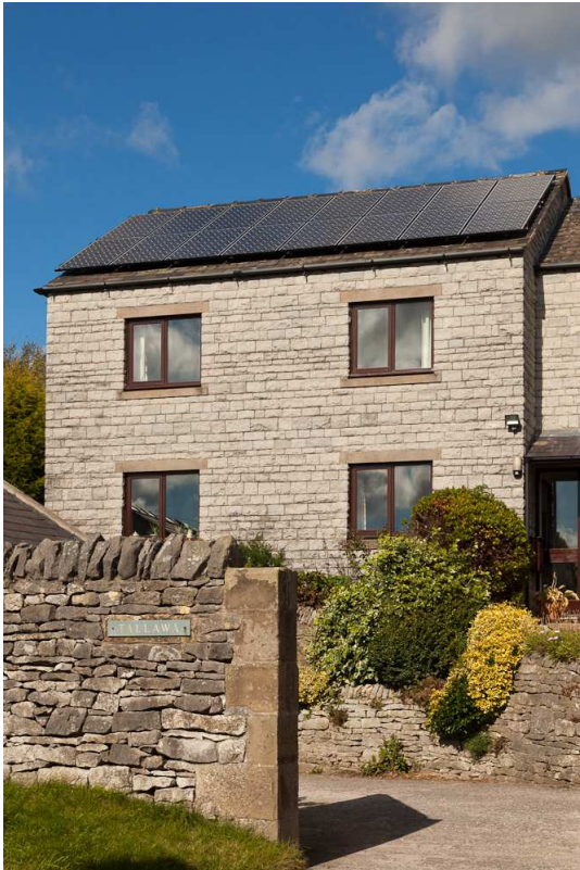
Photo 9. Retrofitted photovoltaics, Over Haddon
