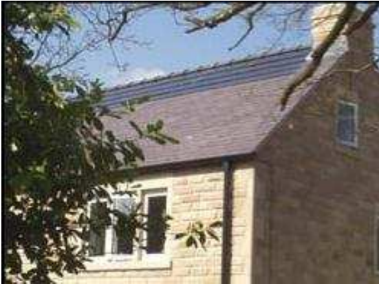
Photo 10. New build replacement dwelling, Curbar with simple arrangement of solar panels below the ridge
