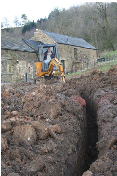
Photo 12. Excavation for Ground Source Heat Pump, Dove Valley Farm
