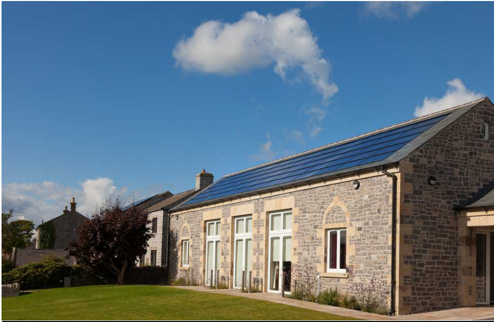
Photo 4. New build village hall, Over Haddon
