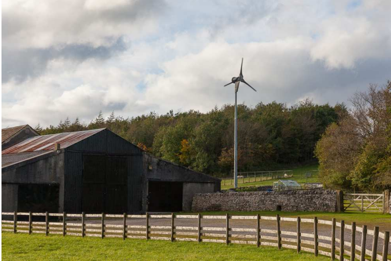
Photo 22. Example of turbine located close to buildings and facing into the prevailing wind
